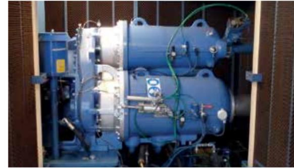
Stork recovered energy from a 430 kW/hour air compressor to heat up process water.
