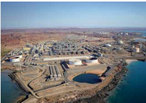
Located 1,260 kilometers (783 miles) north of Perth, Western Australia and covering approximately 200 hectares (494.2 acres), the North West Shelf Project's Karratha Gas Plant includes five LNG processing trains, two domestic gas trains, six condensate stabilization units, three LPG fractionation units, as well as storage and loading facilities for LNG, LPG and condensate. The plant has the capacity to produce 12,000 metric tons of domestic gas per day.
