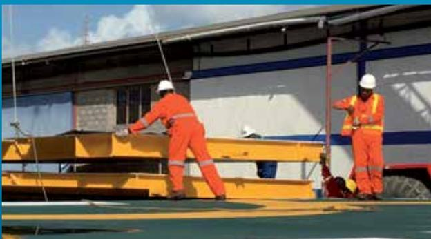
Due to corrosion and rigorous offshore conditions, this helideck was in dire need of replacement. The scope of this job included the construction of a wider superstructure and sub-structure to accommodate a larger chopper, in accordance with the Civil Aviation Authority 437 Standard.
