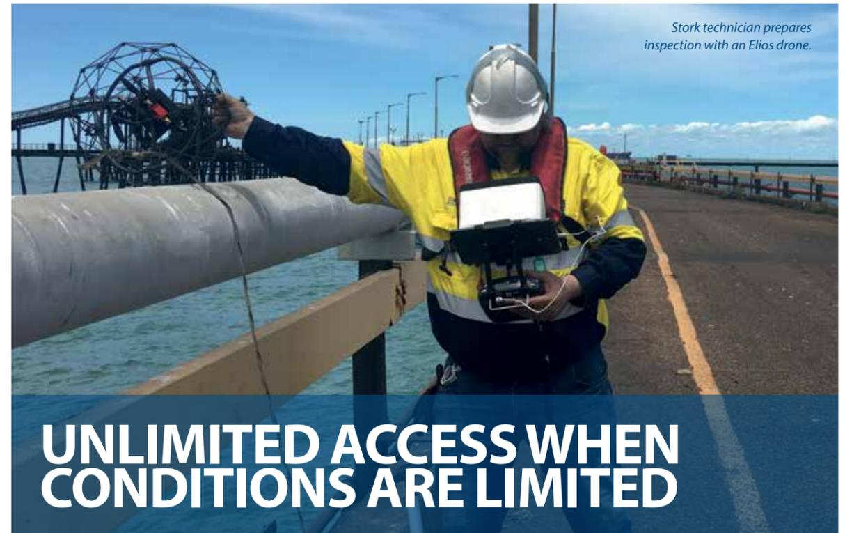
Stork technician prepares inspection with an Elios drone.
