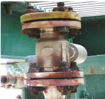
Four Bolt Flange condition prior to workscope
