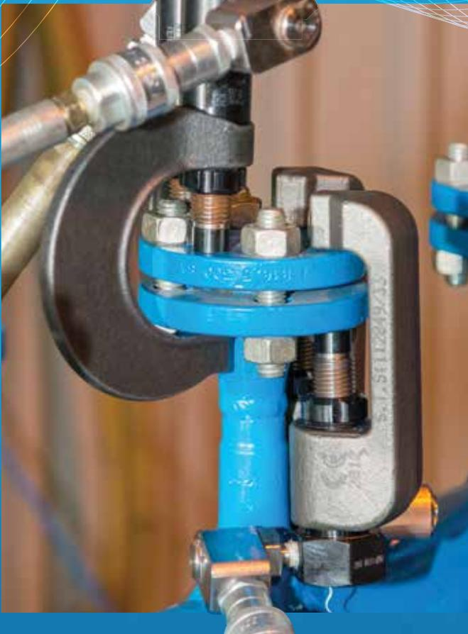
We identified a significant cost, time and safety issue for all offshore clients whereby restrictions on the live hot bolting of 4 bolt flanges forced clients to tackle such systems only during specific shutdowns, - a costly and time consuming activity.
