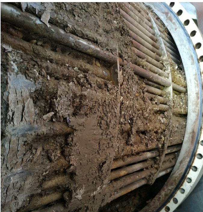
Photo: Before cleaning
