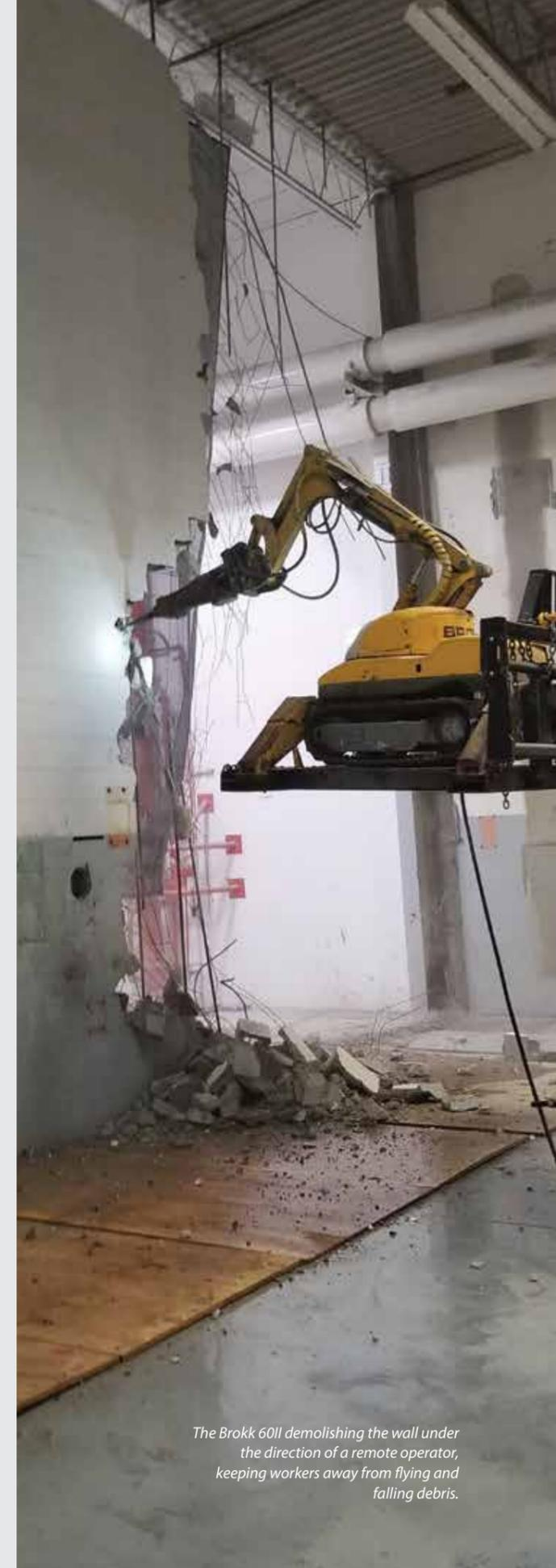
*The Brokk 60II demolishing the wall under the direction of a remote operator, keeping workers away from flying and falling debris.*
