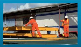
Due to corrosion and rigorous offshore conditions, this helideck was in dire need of replacement. The scope of this job included the construction of a wider superstructure and sub-structure to accommodate a larger chopper, in accordance with the Civil Aviation Authority 437 Standard.
